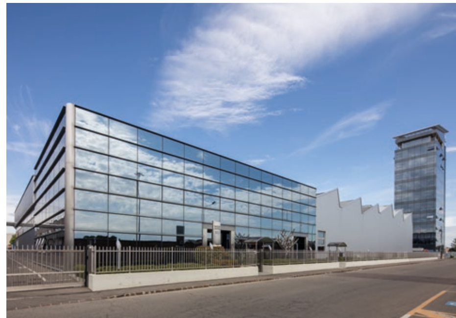
CPC Group Auditorium Modena, Italy
