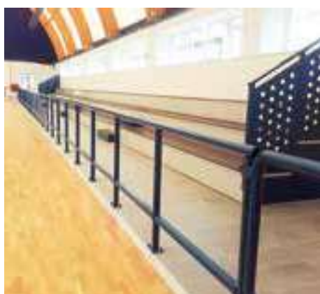
Transenna con montanti, corrimano e barra inferiore. Su bussole o piastre Barrier with uprights, single handrail and lower bar. With ground sockets or plates.
